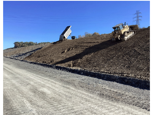
Topsoil placement on slopes at finished grade.
