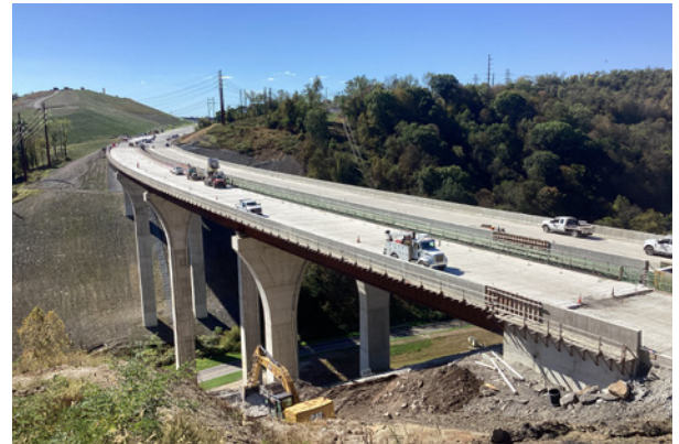
Bridges over Coal Valley Road - construction progress.
