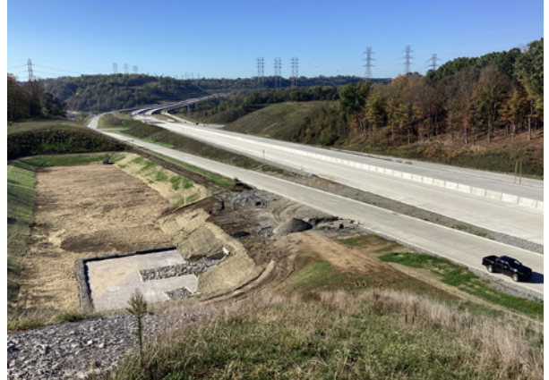
New highway looking south to Jefferson Boulevard interchange.
