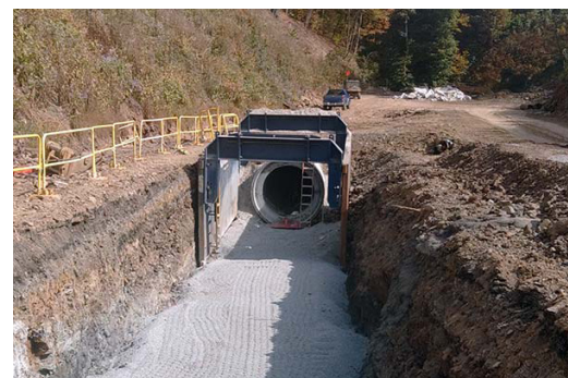
72 inch reinforced concrete pipe installation near former Millers Road.
