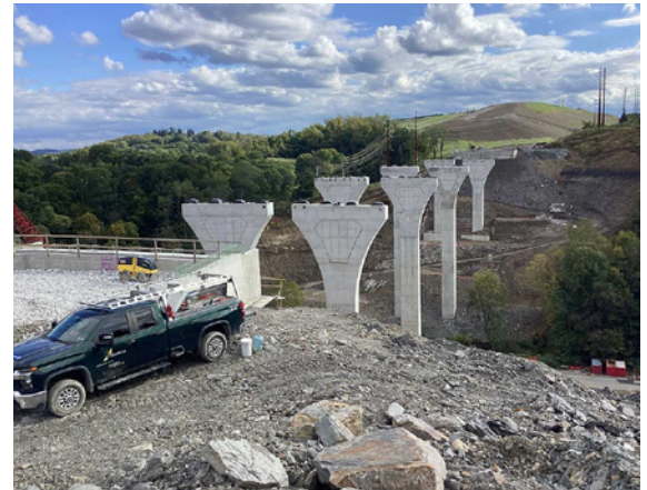
Bridges over Coal Valley Road construction progress.
