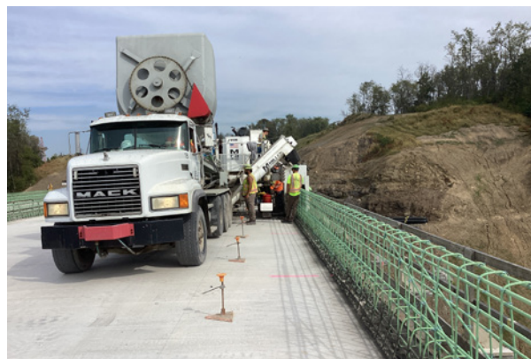
Concrete bridge parapet placement - bridges over Coal Valley Road.
