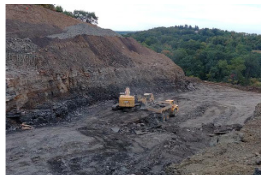
Excavation work near Coal Valley Road.
