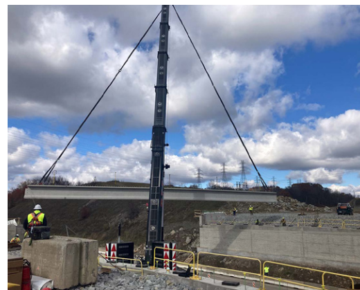
First beam for the new highway being erected over Jefferson Boulevard.
