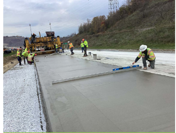
Long life concrete pavement paving operation.
