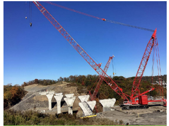
Crane preparation for steel girder erection at bridges over Coal Valley.
