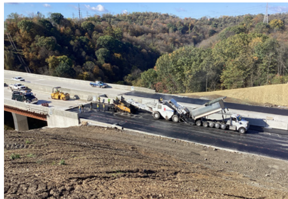
Bridges over Coal Valley Road - transition asphalt paving.
