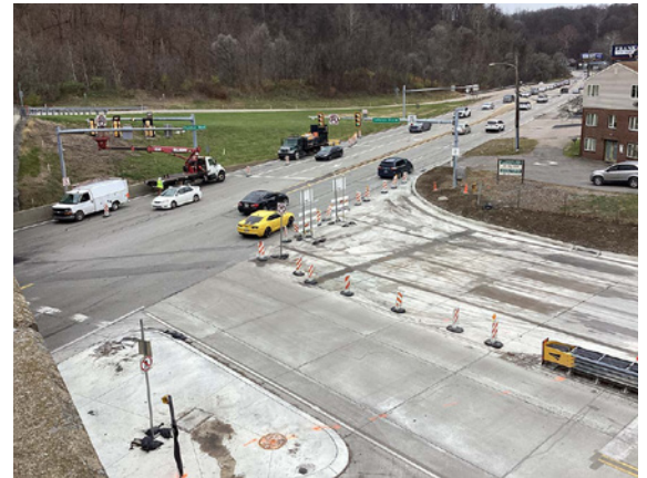
SR-51-Jefferson Boulevard intersection nearing completion.
