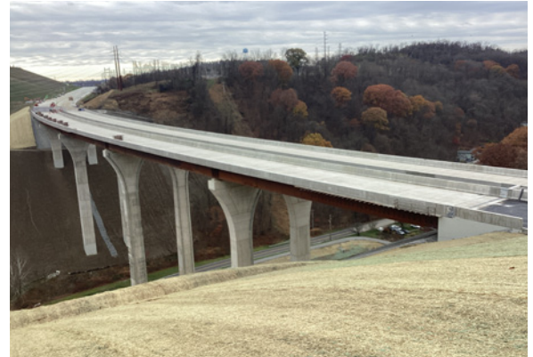
Bridges over Coal Valley Road - near completion.
