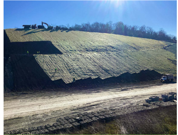
Seeding and erosion mat installation on completed cut slope
