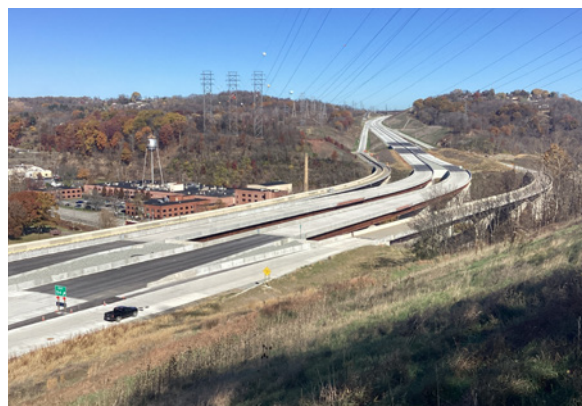
Bridges over SR51- near completion.
