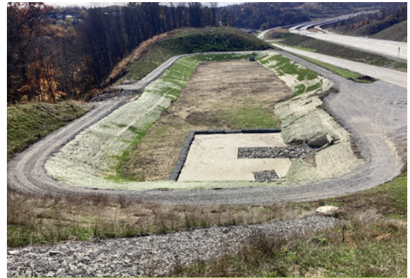
Stormwater management pond complete.
