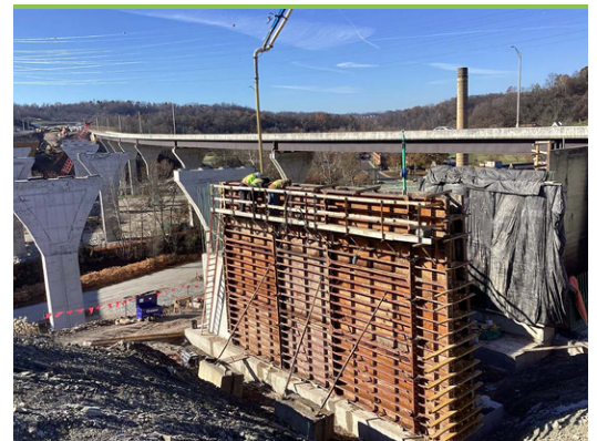
A concrete wall is being constructed for northbound bridge over SR51.
