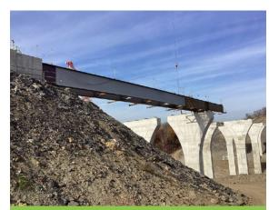
Steel erection for bridge over Coal Valley Road.
