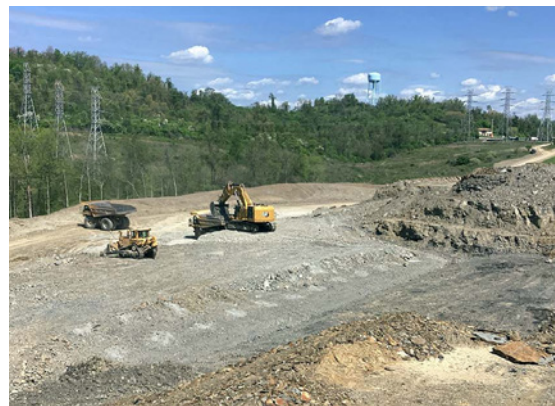
Bulk excavation near SR 885.
