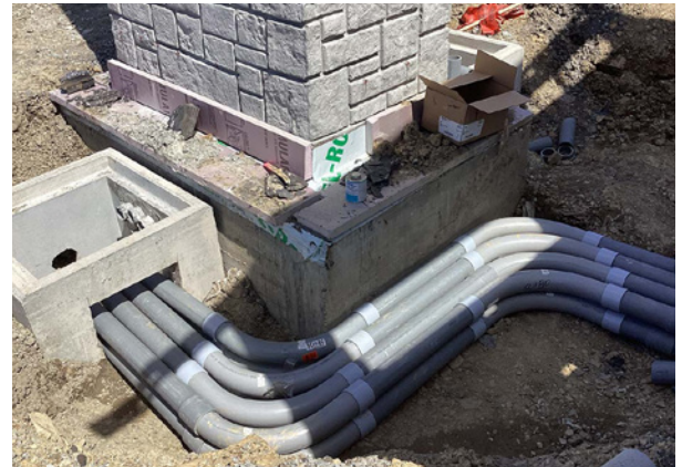
Conduit installation for over the road tolling equipment.
