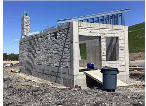
Roof installation for tolling building.
