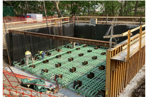
MF-401 Pier 4 Footing.
