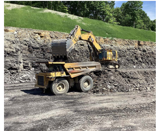
Excavation south of SR-885.
