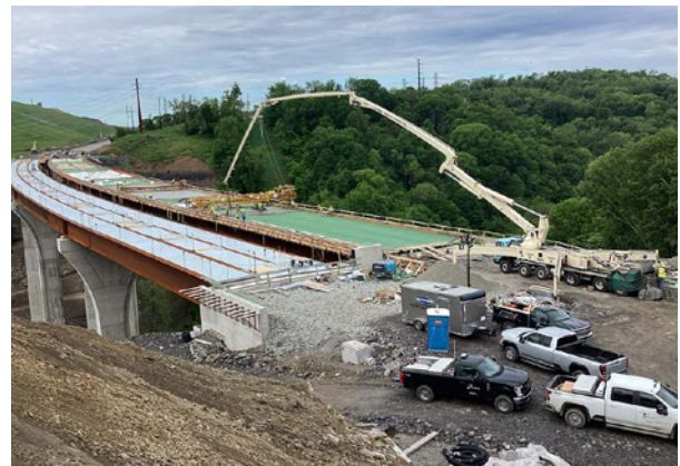
Concrete deck placement for bridge over Coal Valley Road.
