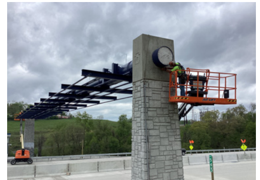
Over the road tolling gantry installation.
