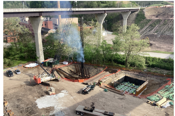
Bridge 401 Pier Pile Driving
