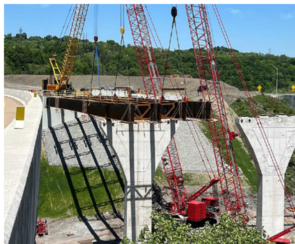
MF-401 Span 6 Erection (bridge over SR51).
