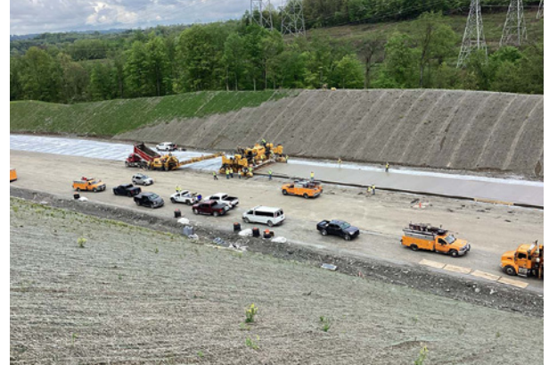
Concrete paving for PTC 43 northbound travel lanes.
