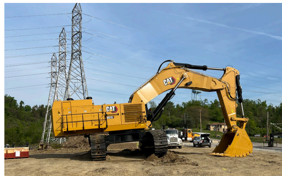
Large Excavator Being Assembled for Bulk Excavation
