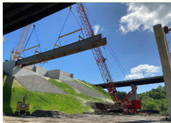
First beams being erected for bridge to span SR 51.
