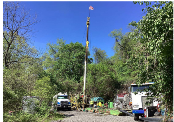
Gas well plugging on future Section 53B1A.
