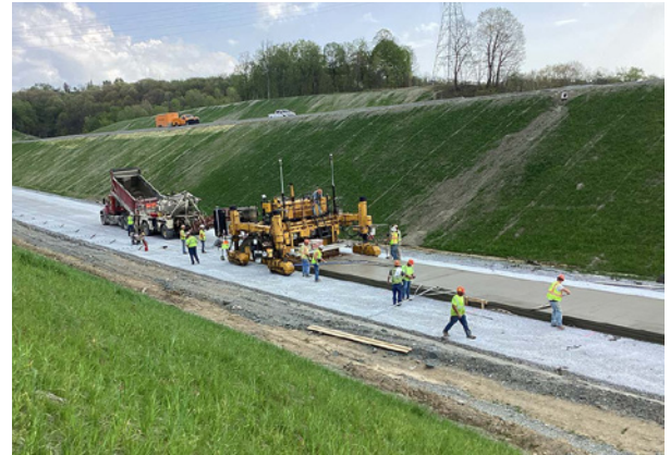
Concrete paving for PTC 43 southbound off ramp at Jefferson Boulevard.
