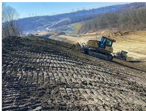
Topsoil placement on finished slope.
