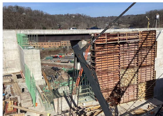
Construction of southbound PTC 43 bridge abutment over SR 51.
