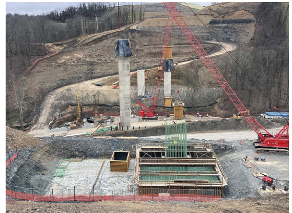
Pier construction for bridges over Coal Valley Road.
