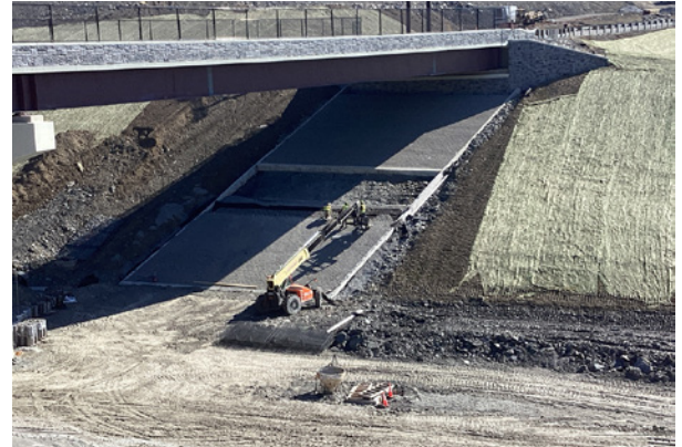
Construction of articulating cellular block slope wall for SR 885 bridge.
