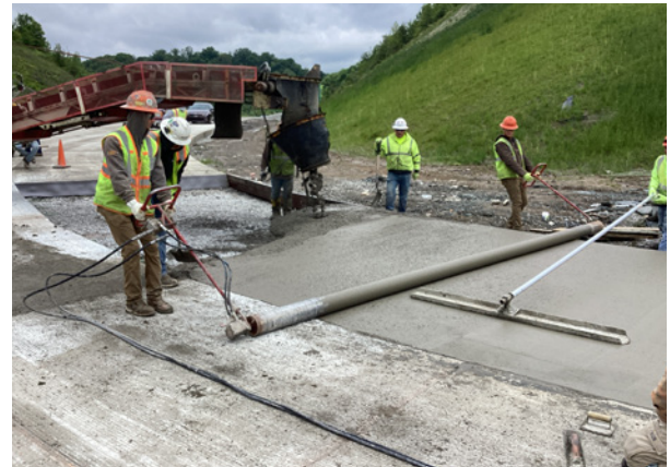
Concrete roadway placement - Future 43 southbound on ramp.
