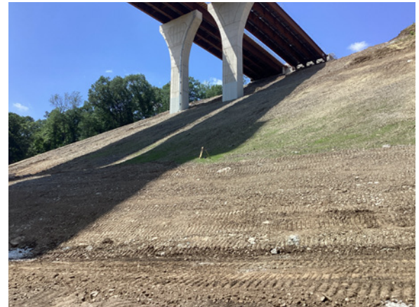
Grading final slope under Coal Valley Road bridges.
