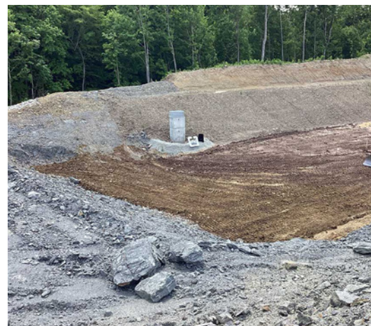
Sediment basin construction.
