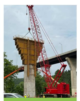
Crews are forming a cap on a pier that will help support the bridge over S.R. 51.
