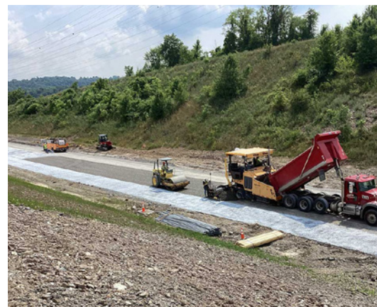
Reconstructing Jefferson Avenue PTC-43 Southbound.
