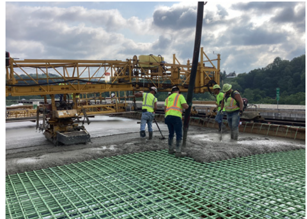
Concrete bridge deck placement for bridge over SR51.
