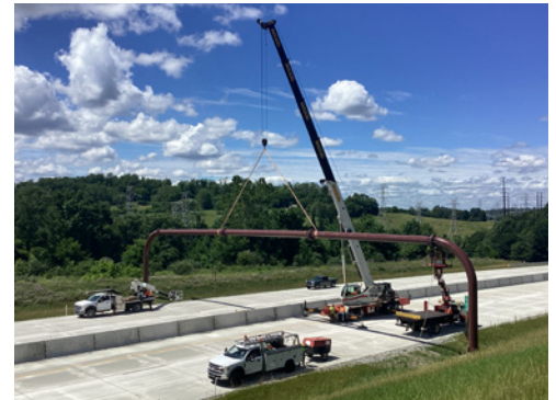
Overhead sign installation.
