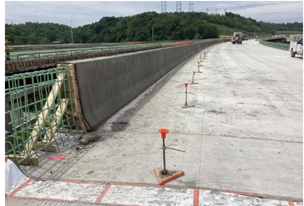
Bridge parapet construction on bridge over SR-51.
