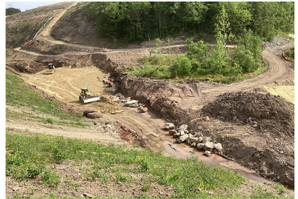
Undercut and Backfill for Culvert A
