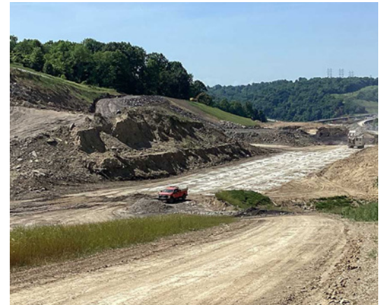
Drilling for blasting operation
