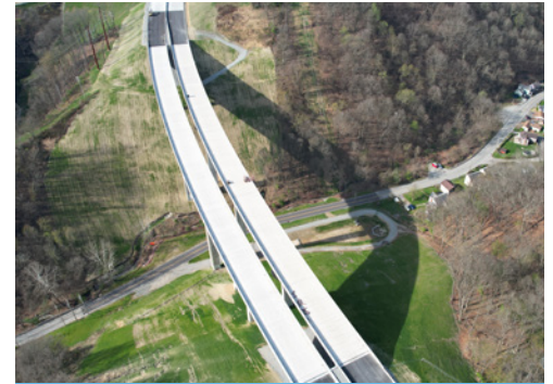
Bridges over Coal Valley Road.
