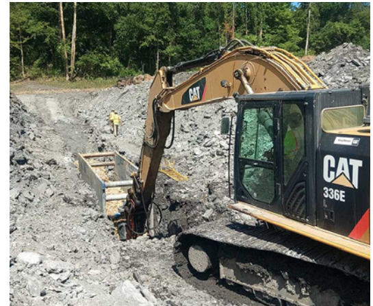
Excavation for drainage.
