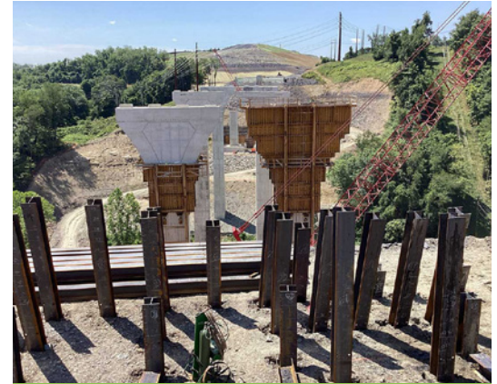
Bridges over Coal Valley Road construction progress.
