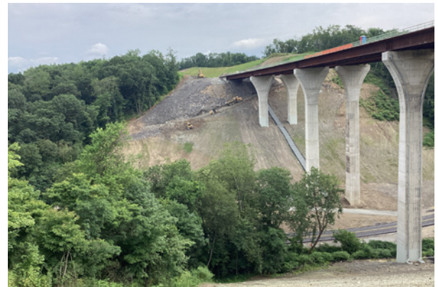
Slope construction under the Coal Valley Road bridges.
