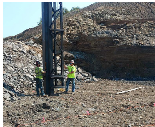
MF 405 abutment 2 pile testing (bridge over Coal Valley Road).
