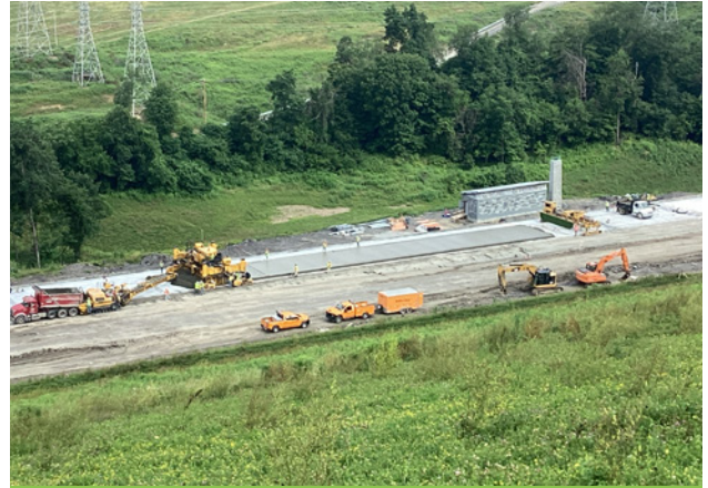
Roadway concrete paving near future toll facility.
