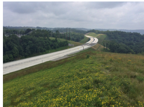
New highway looking north across Coal Valley Road.
