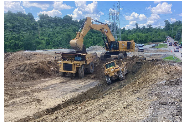
Bulk Excavation Occuring Near SR 885 Utilizing Large Off-Road Trucks.
