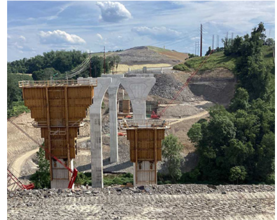
Bridges over Coal Valley Road construction progress.
