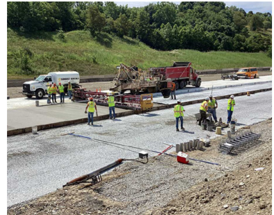
PTC-43 Southbound long life concrete pavement operation.
